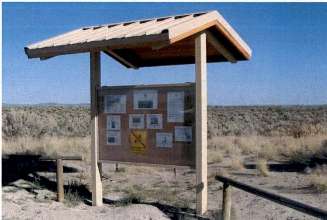
Figure 7. Sample kiosk installed with excavated post holes (image source: naturalstructures.com).
