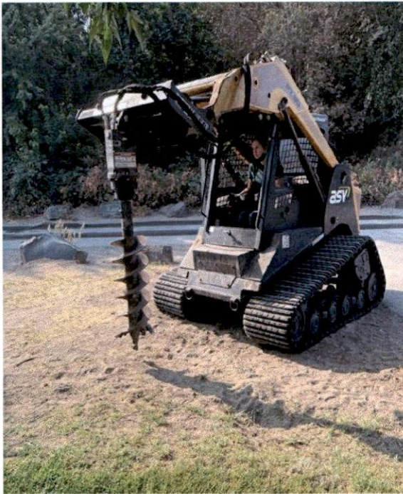
Figure 13. Boat Launch API. Proposed kiosk location. View to the southwest.
