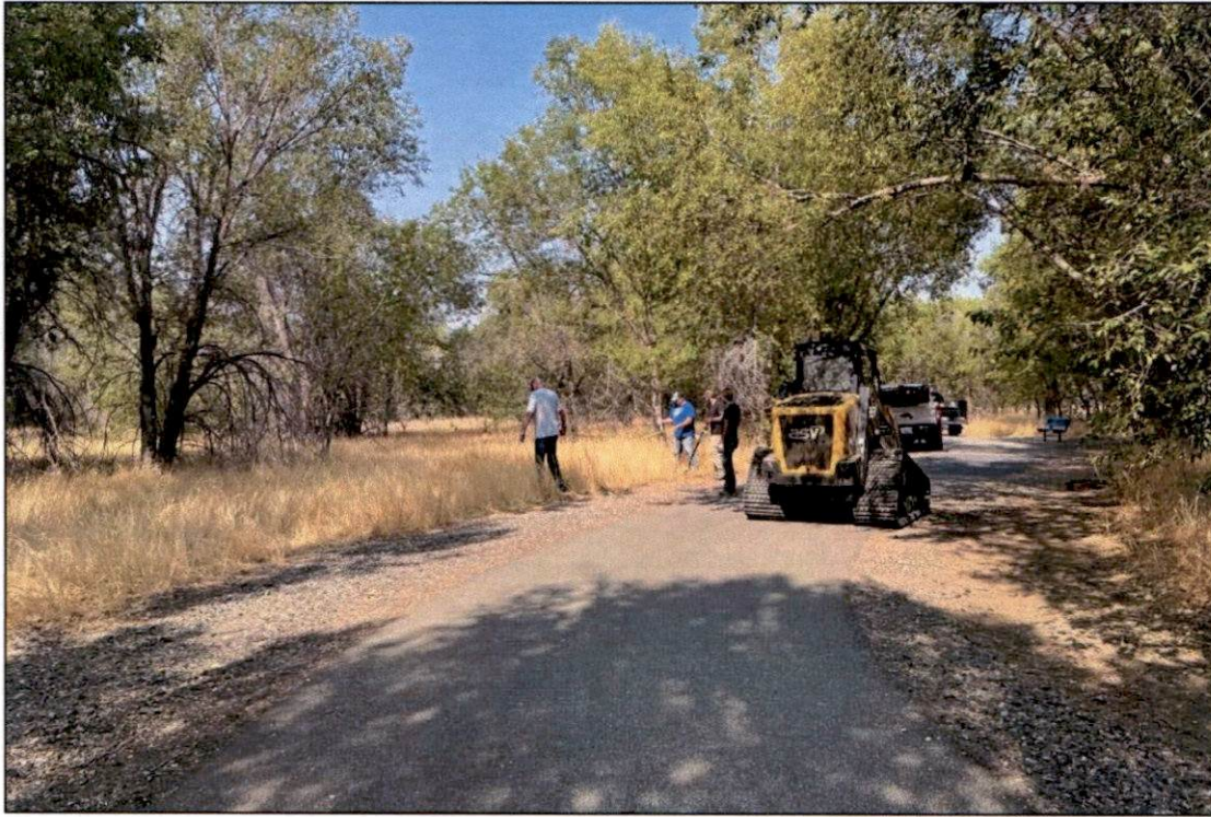
Figure 2. Benton City's 14th Street API at the proposed location of Kiosk 2. View to the west.
