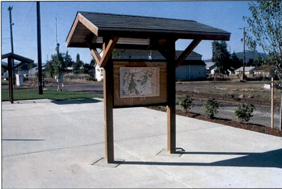
Figure 8. Sample kiosk installed using a concrete pad (image source: naturalstructures.com).
